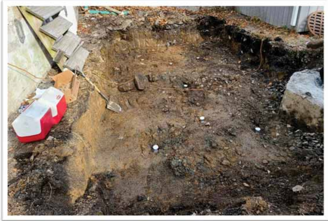
Excavation 1 – Looking West
