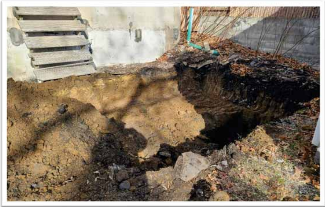
Excavation 1 – Looking Northwest
