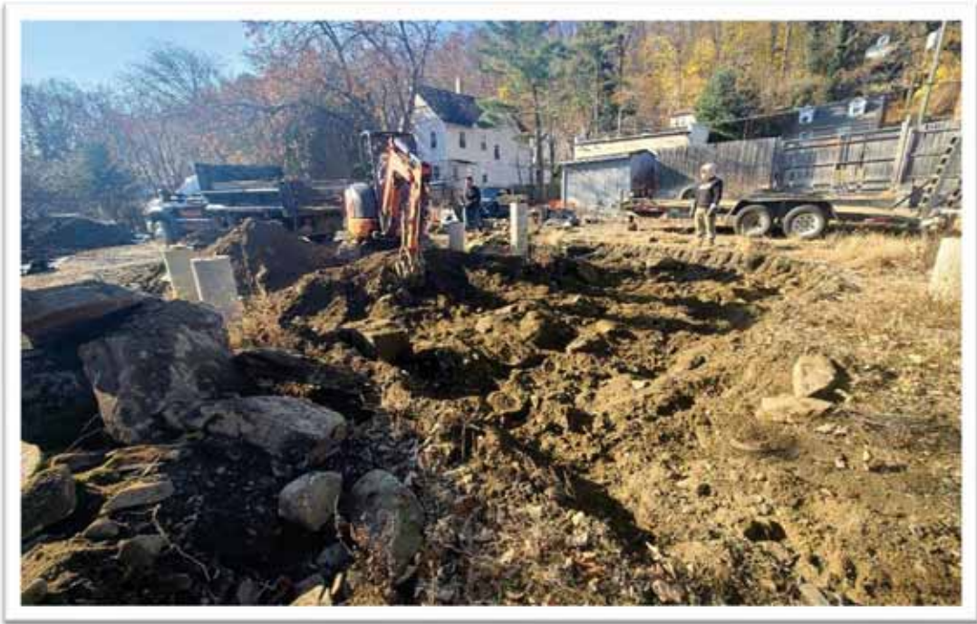
Excavation 3 – Looking Northwest
