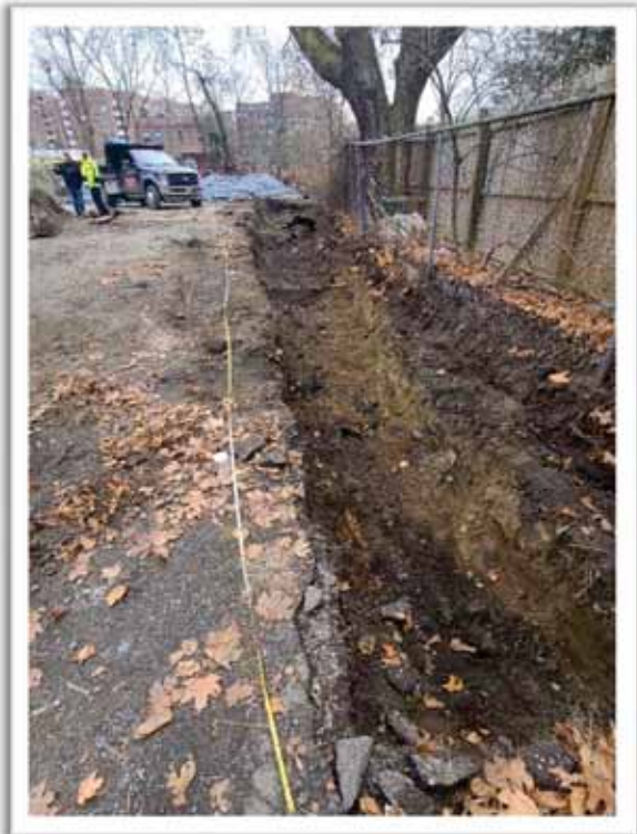
Excavation 2 – Looking South
