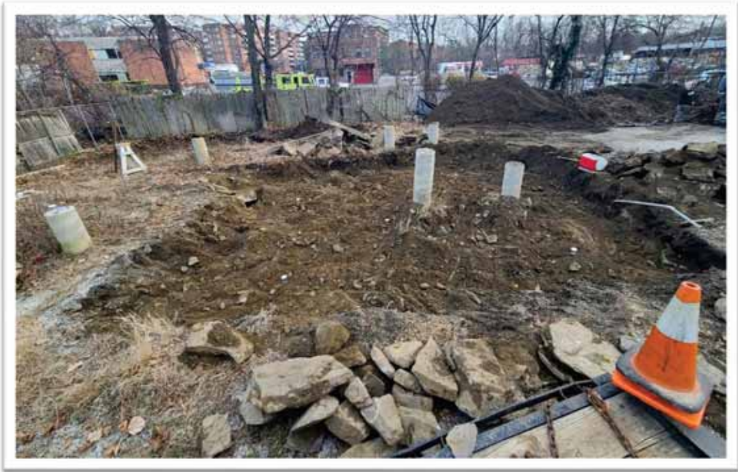
Excavation 3 – Looking West
