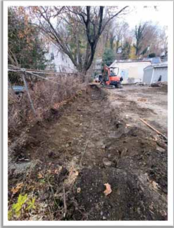
Excavation 2 – Looking North
